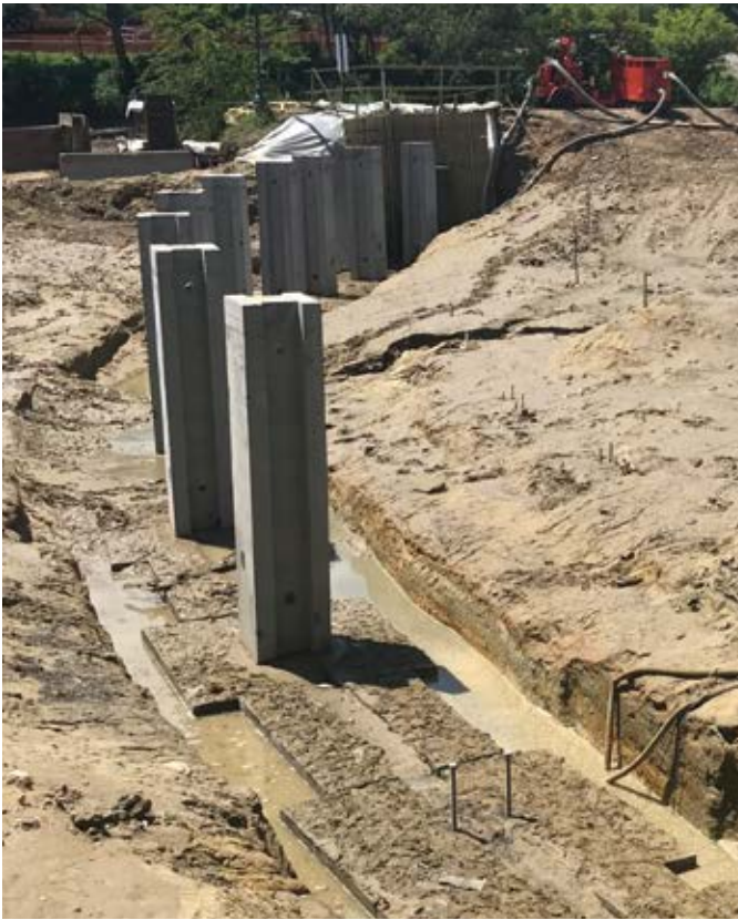
Using precast concrete products was more cost- and time-effective to construct the base for the bridge thanks to its ease of installation.
