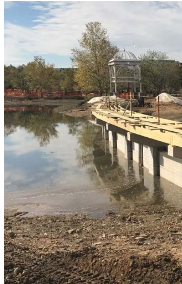
Using precast concrete products was more cost- and time-effective to construct the base for the bridge thanks to its ease of installation.
