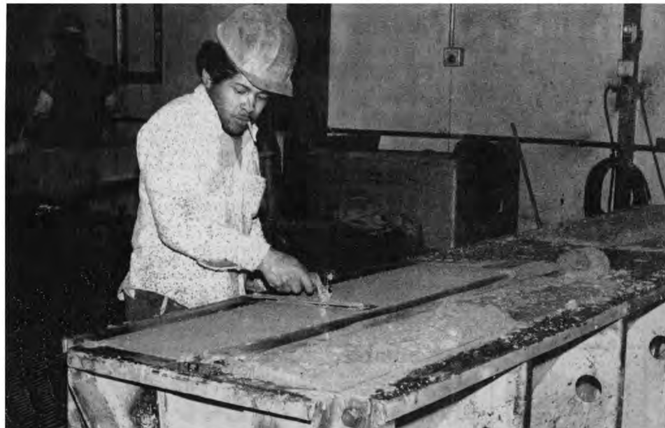
THE FINAL STEP in barrier production is performed by Andrew Washington of Casanova at the Midland plant.
