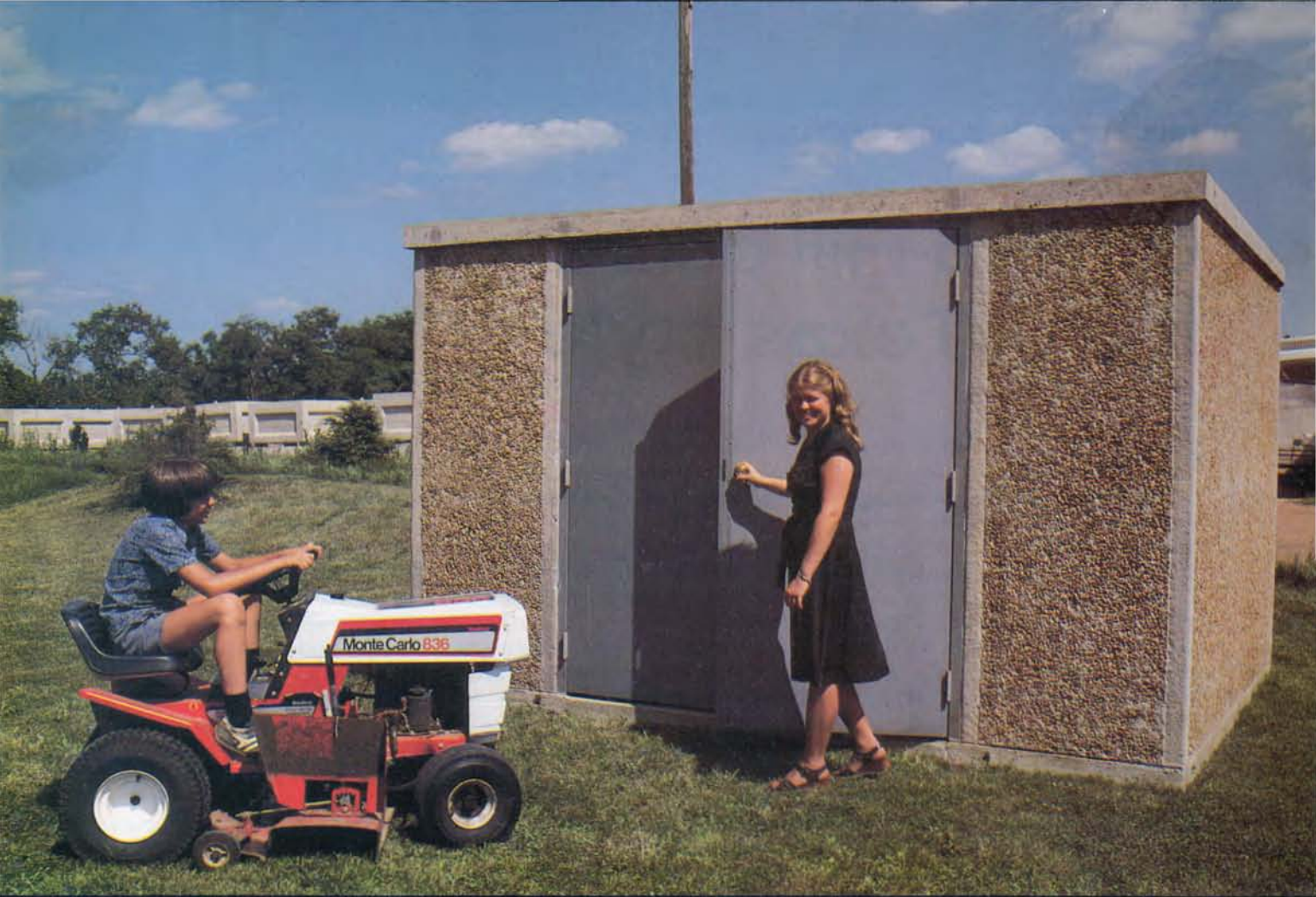
Exterior walls of this all-purpose structure have exposed aggregate finish.
