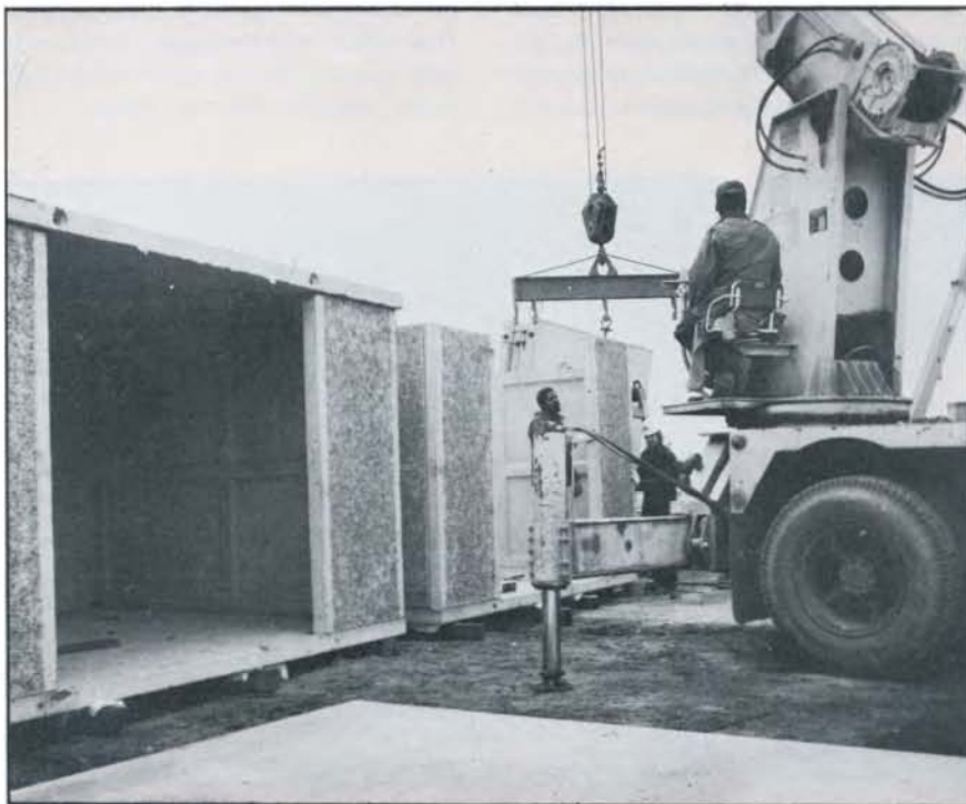
Buildings are assembled at the plant with seven panels.
