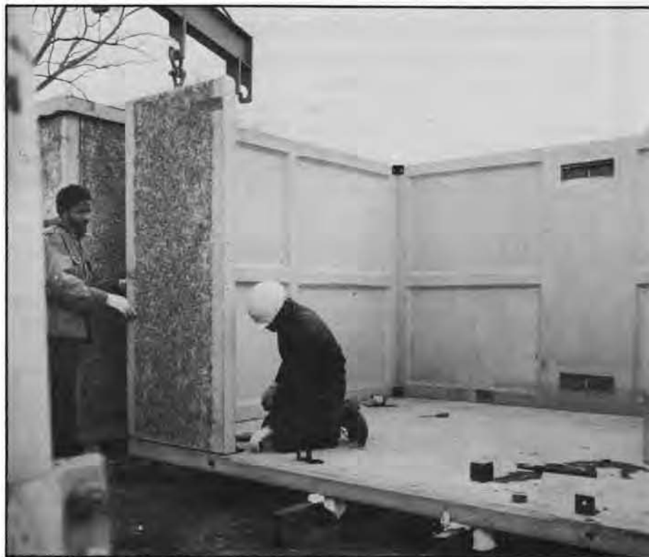
Recessed pattern of interior surface saves weight, adds to appearance.
