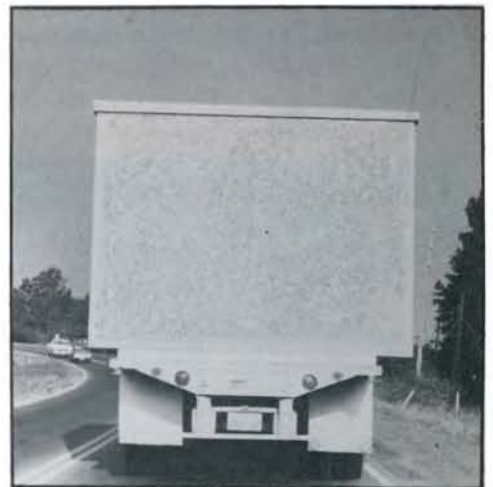
Loaded on a trailer, the 20,000-lb. building heads for installation site.
