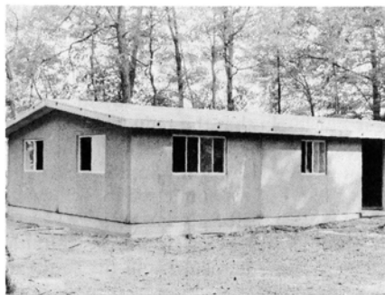
The Smith Company hopes precast concrete houses are the future.
