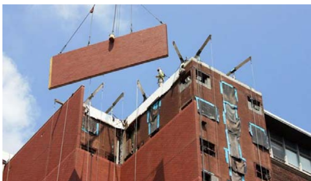
Slenderwall, a pre-cast engineered concrete panel used in building construction, will be made at Smith-Midland's new manufacturing facility in Hopkins. (Photo/Provided)
