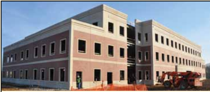
Office of the Chief of the Army Reserves (OCAR) Ft. Belvoir, VA: architectural precast - 33,202 sf 100% complete; Client: Hensel-Phelps Construction Co.
