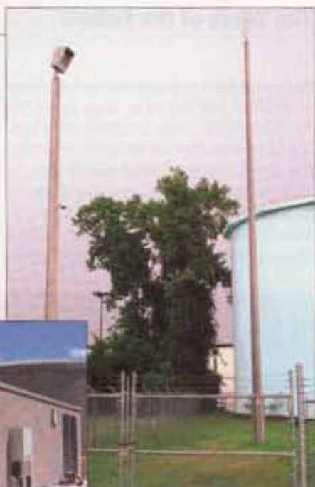
One Lonestar Prestress 35-foot tall prestressed concrete camera pole with light and one 70-foot tall antenna pole installed at a Houston groundwater facility.
