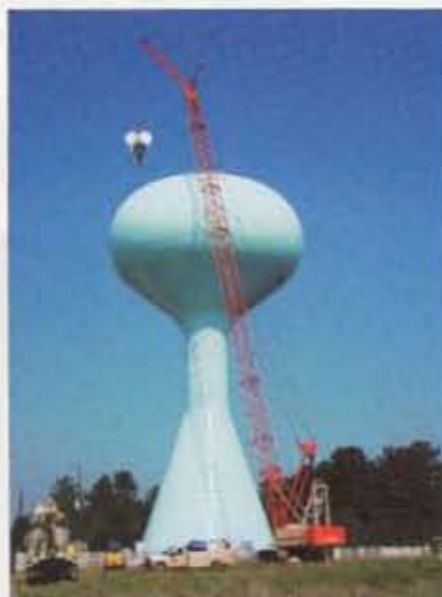
Boyer Inc's 100-ton crane placing a fully dressed antenna pod atop a water tower in Houston.
