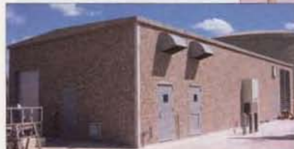
An example of a Lonestar Prestress Easi-Span 30x70x15 (clear span) site-erect precast concrete buildings in Friendswood, TX.
