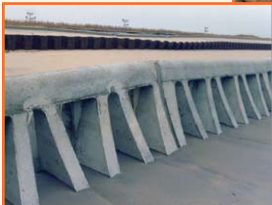
Installation on Wallop's Island
