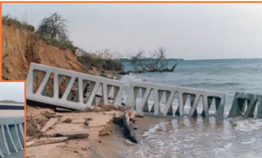
Beach Prisms™ installation in Stevensville, MD
