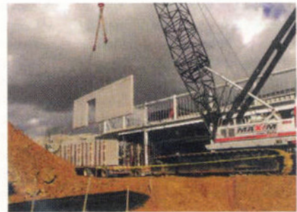
Smith-Midland Corporation provided dramatic and cost-effective precast panels for Virginia Tech's new basketball facility.
