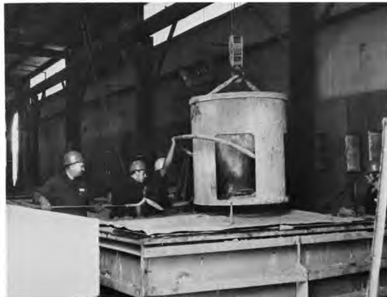
Bucket handled by bridge crane holds concrete for big utility vault pour.
