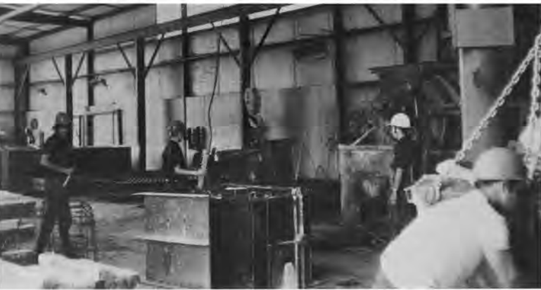
These forms are used to cast covers for smaller utility vaults.
