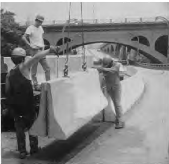
Biggest order to date were these pre-cast median barriers installed in nation's Capital.
