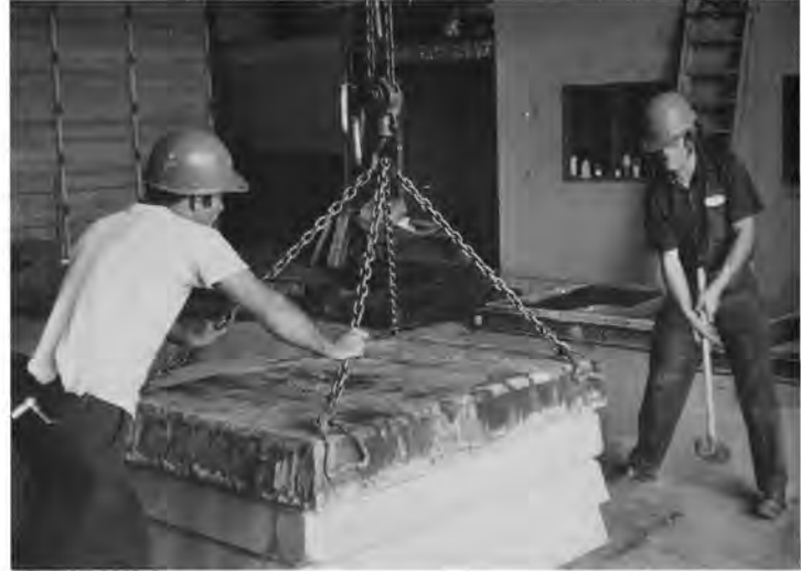
These forms are used to cast covers for smaller utility vaults.
