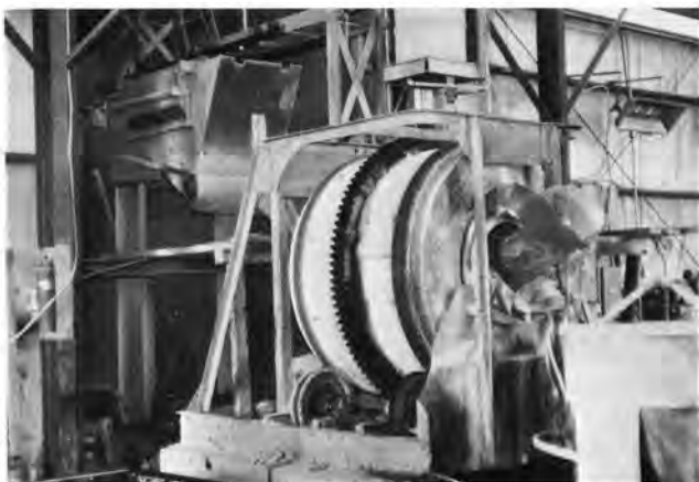
Concrete mixer (1 yd.) is fed by hand-pushed hopper which is charged from bins.
