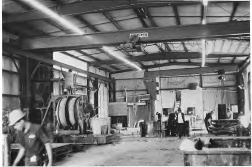
Overall view of main production area.
