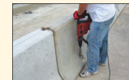
Drilling hole
