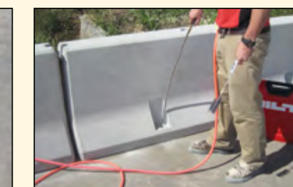
Cleaning hole with air and brushing
