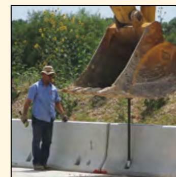
Pins installed - 3 minutes each
