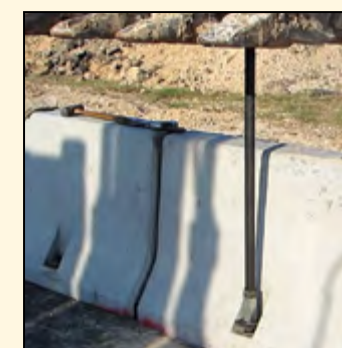
Pin installed
