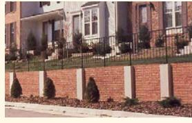
**HIGHWAY** - Sound wall is widely recognized and accepted as an effective sound barrier system. Standard highway sections measure 16', 20', or 24' from center to center and can be manufactured to heights up to and exceeding 30'.
