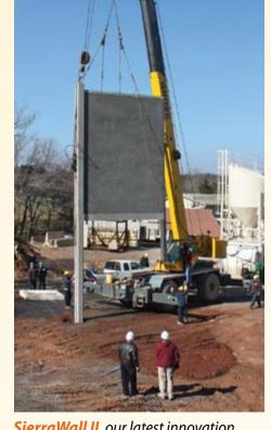
SierraWall II, our latest innovation. A one-piece post & panel sound wall, designed to save our customers on both manufacturing and installation costs.
