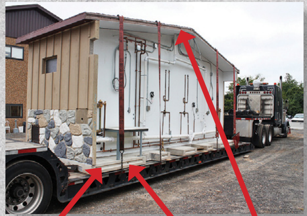
Grout keyways Post-tension conduits, floor and roof
