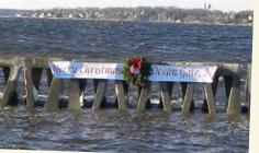
January 14, 2014 – Adorned with a sign that said, "Merry Christmas Ocean Gate," 35 precast beach prisms recently made their New Jersey debut. Manufactured from precast concrete, the prisms are constructed with cut-through holes that allow the ocean to flow naturally without removing sand from beach.
