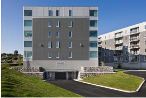
Luxembourg III Apartments, Quebec
