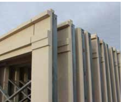
The goal for the Cliffside Park Towne Center project was to create the feel of a classic limestone building with a modern twist.
