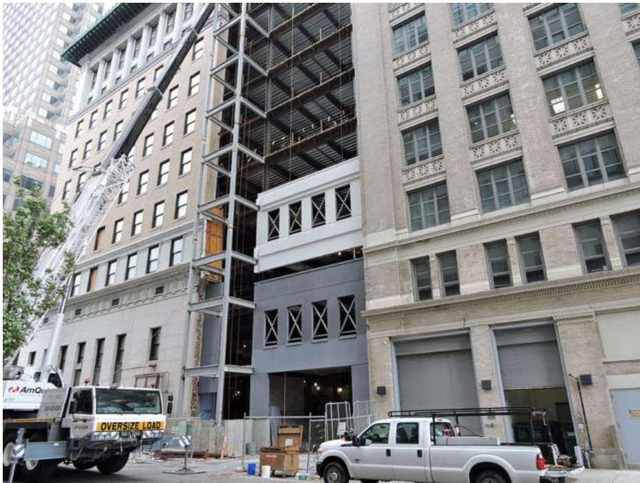
(Hyatt House construction, courtesy Easi-Set Worldwide)
