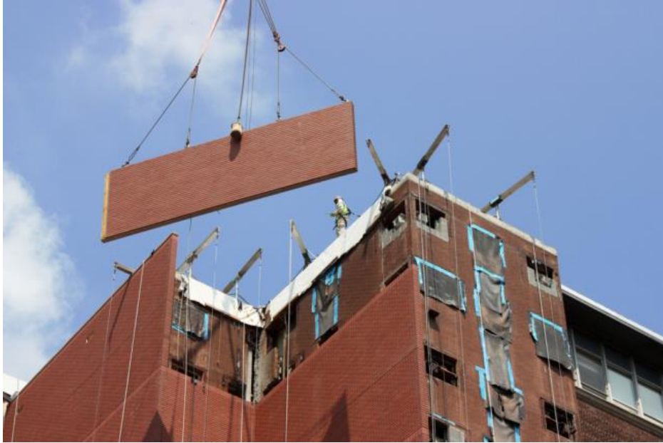
(Johns Hopkins re-cladding, courtesy Easi-Set Worldwide)
