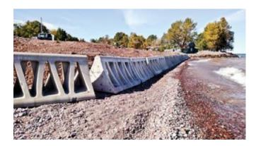
The Beach Prisms installed near the mouth of Oman's Creek at Little Girl's Point Thursday have built-in parabolic curves that break the energy of waves traveling through them, designed to prevent erosion of the section of lakeshore.
