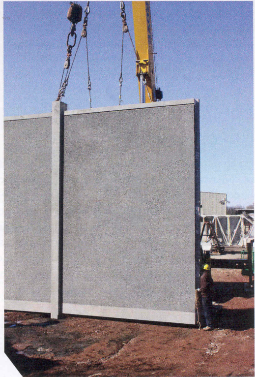
The new Sierra Wall II from Smith-Midland is an update to the one-piece precast concrete column and sound panel system. Courtesy of Dale Neal.
