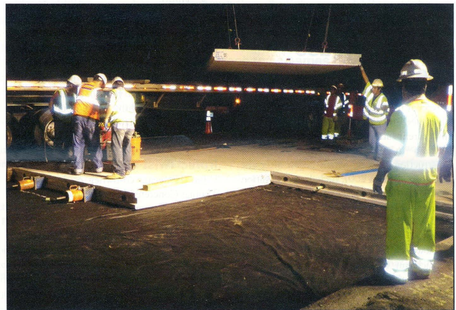
Workers place the 306 slabs of precast/prestressed concrete that are finished with a light broom finish.
