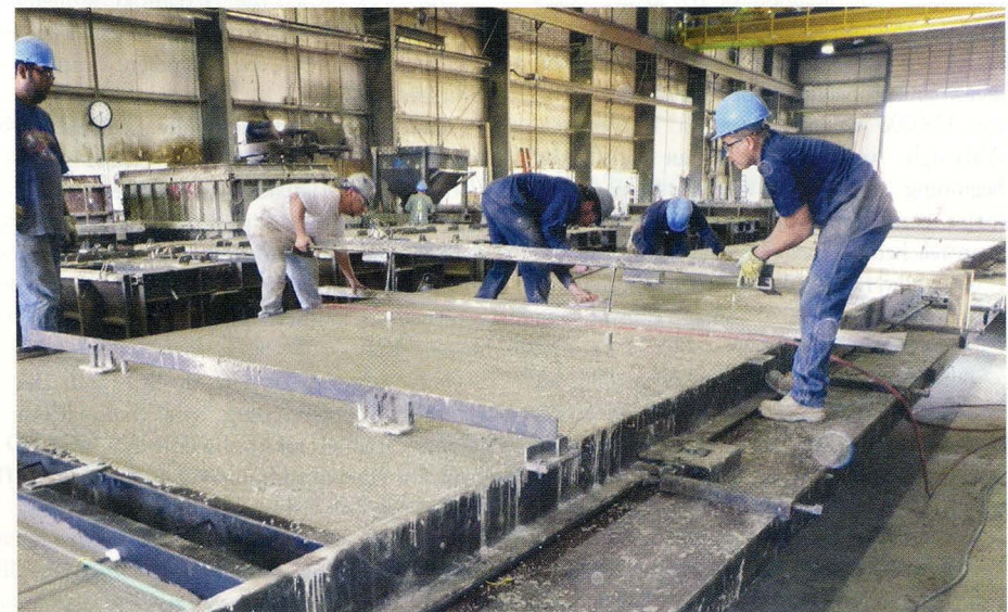
The slabs are manufactured in Smith-Midland's Virginia plant.
