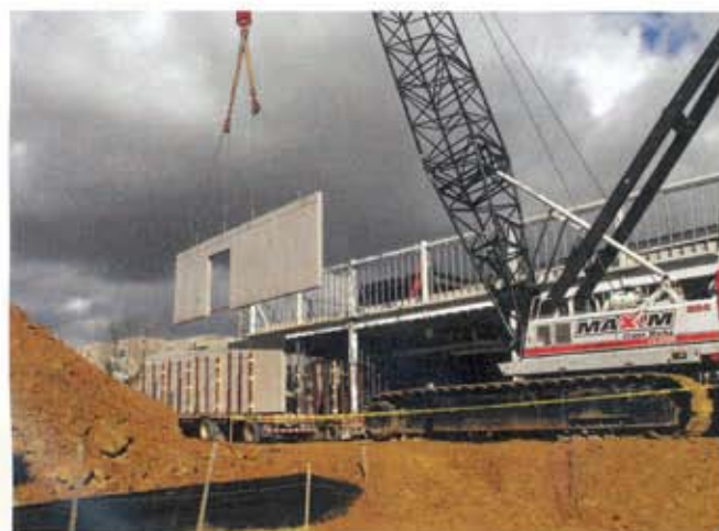
Baltimore-based EE Marr Erectors uses a 200-ton Link-Belt LS-248H to lift the precast panels into place.
