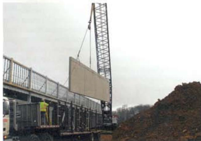
Baltimore-based EE Marr Erectors uses a 200-ton Link-Belt LS-248H to lift the precast panels into place.
