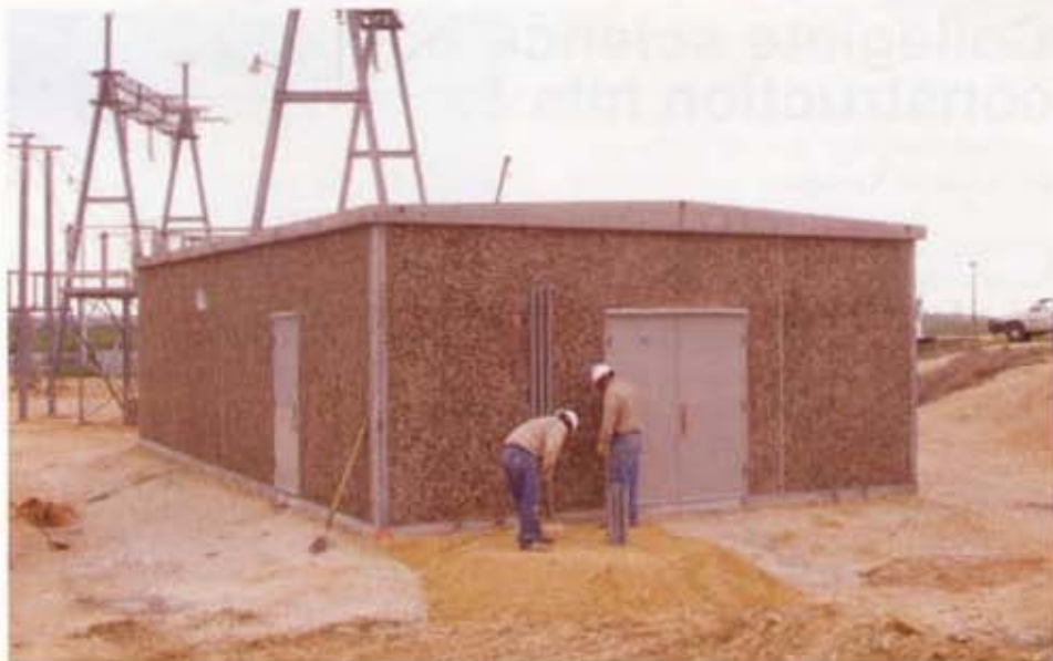
New Braunfels Utility chooses Lonestar Prestress Manufacturing's Easi-Set precast concrete buildings, engineered to withstand 140 mph winds, to house SCADA equipment and other vital infrastructure at local substations currently being overhauled.
