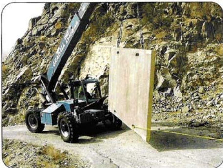
Precast concrete building panels manufactured at Rockway Precast's Las Vegas, Nev., plant had to be transported individually up the remote access road and assembled at the site.
